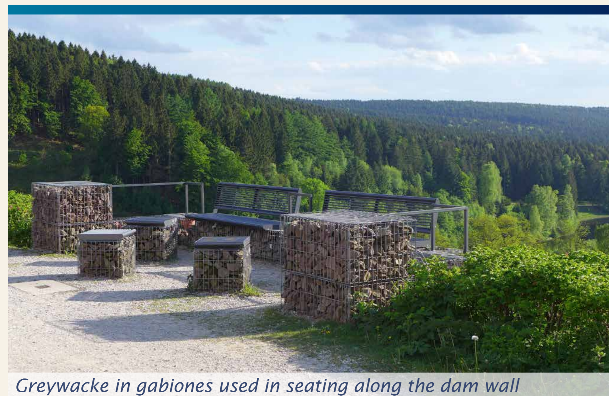
Greywacke used as building material, Wasserläufer Pond, near Clausthal
