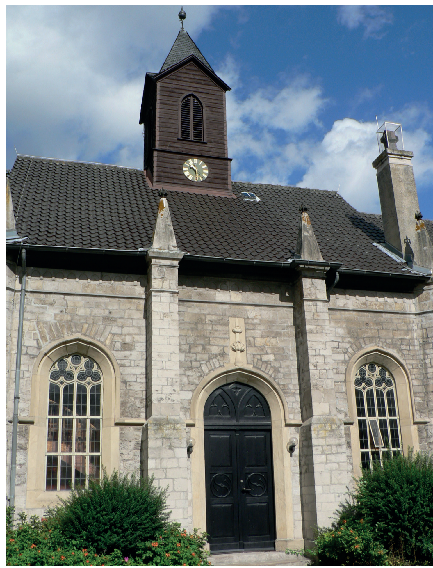
Neubau der St. Antonius-Kapelle (Mitte 19. Jh.), Baustein Dolomit Reconstructed Chapel of St. Anthony (mid-19th century), dolomite stonework
